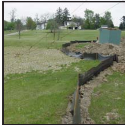
Silt fence installed to protect adjacent property from sediment runoff.
