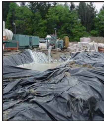
A brine pit collecting fluids pumped from well drilling activities.
